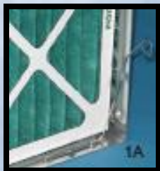
Photo 1A: 2" pleated filter with C-70 fastener.
