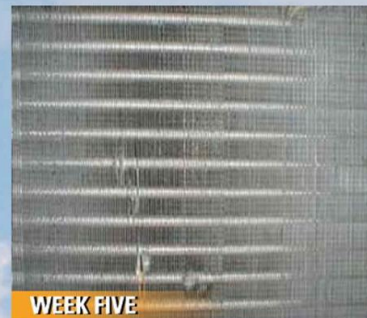
Before and after pictures show fouled coils returned to as-built capacity.
